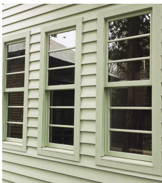
Figure 2. The double hang windows after renovation
