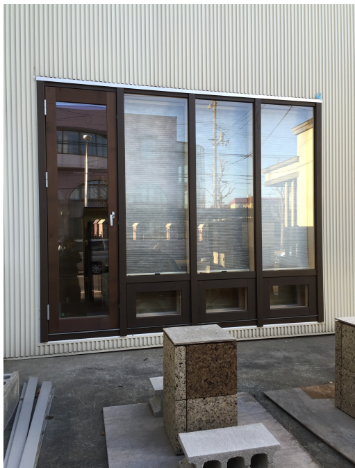
Figure.5 TMW window just installation on the building
