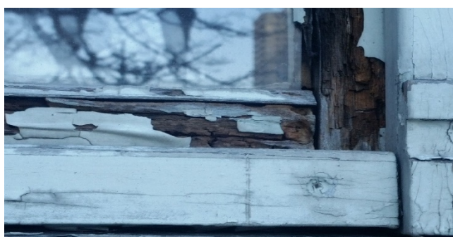
Figure 3 Decayed window frame
