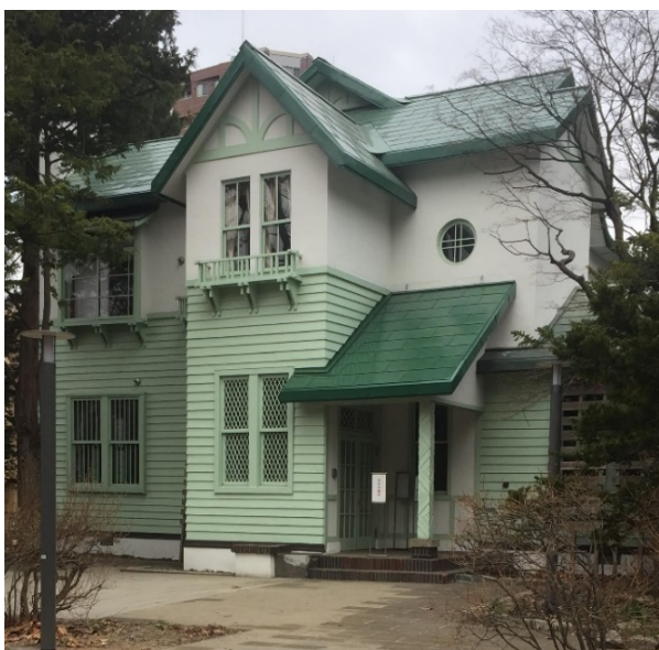
Figure 1. After renovation of old Mitsubishi kougyou dormitory and old Nagayama house.
