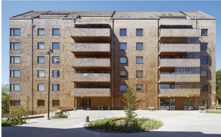
Multi-storey building, Sundbyberg, Sweden.
