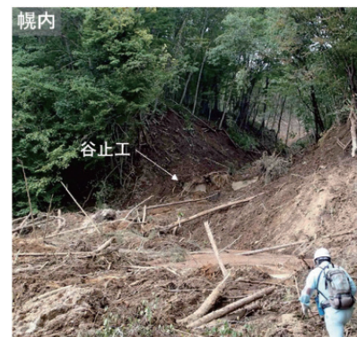
図-11 谷出口の土砂氾濫、地形、谷止工(幌内地区) Fig. 11 Sediment flooding, landform and check dam at an outlet of a creek
