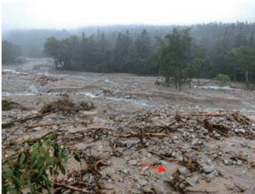
写真-5 1号砂防ダムの土砂・流木の堆積状況 Photo 5 Sediment and drift woods at No.1 sabo dam
